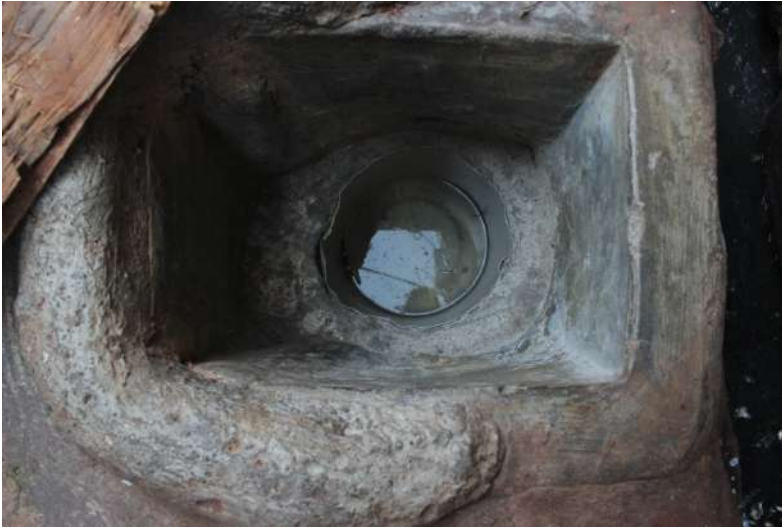
Fig. 27 The pit on the road that stores drinking water for the residents
