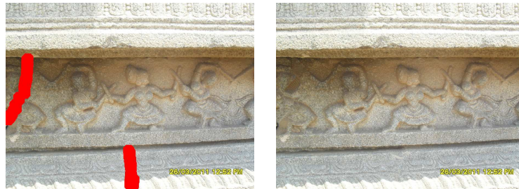
(a) Input image I overlaid with the crack detected in I_g shown in red color (b) Inpainted version of I using the region detected in I_g in red color
