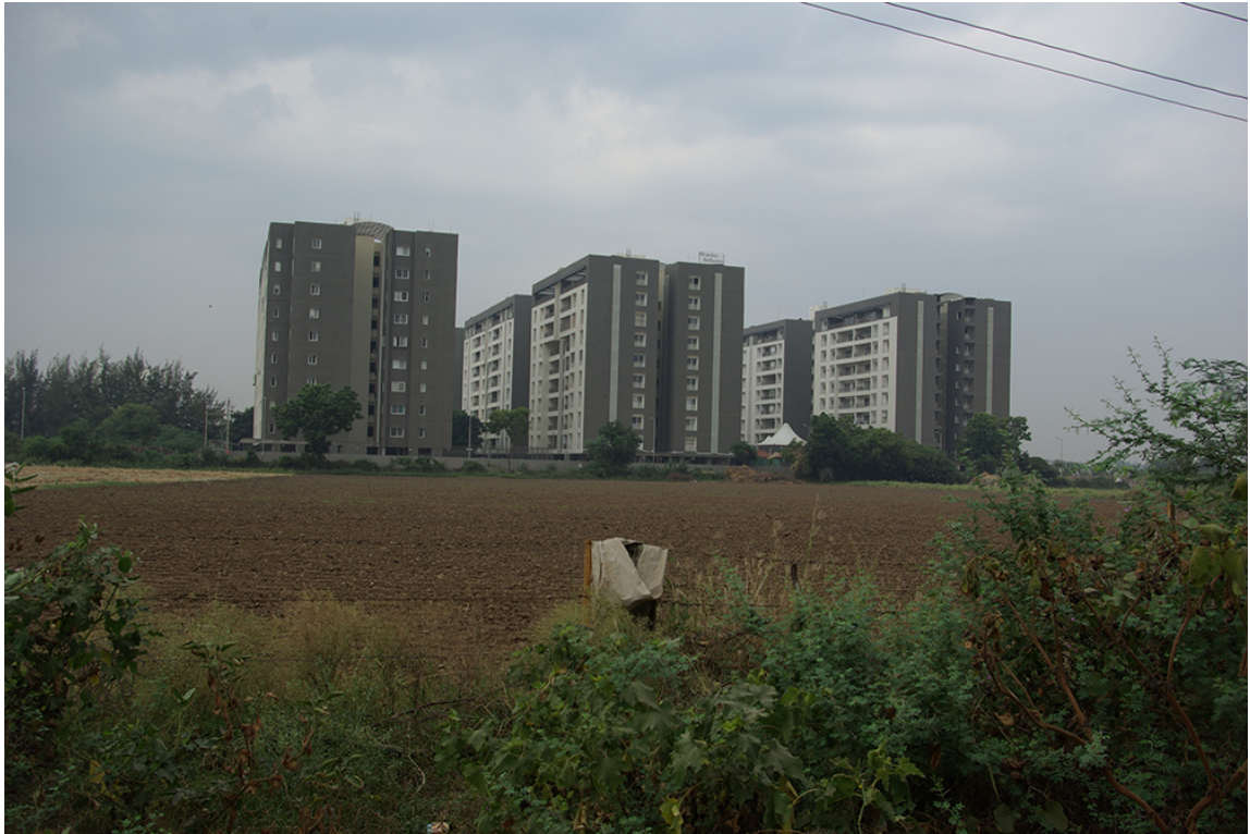
Figure 9.5: New apartment block in Tandalja-Vasna
